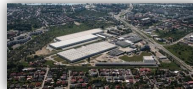
Distribution Park, Wrocław
